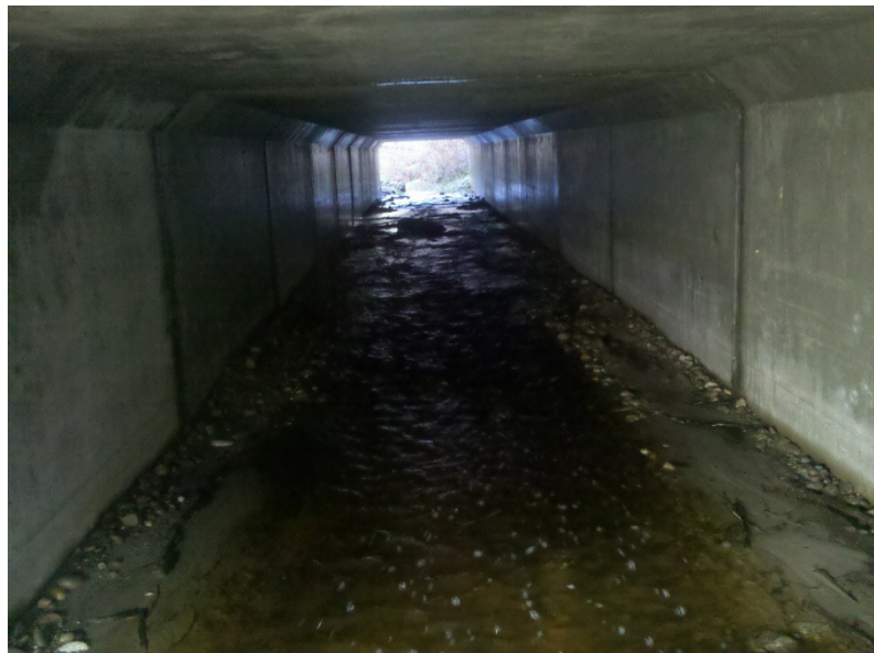
(Above; Culvert under Hood Canal Dr.)
